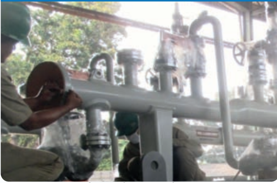
PIG LAUNCHER & RECEIVER
